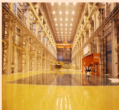
Pressurised Transformer Assembly Bay
