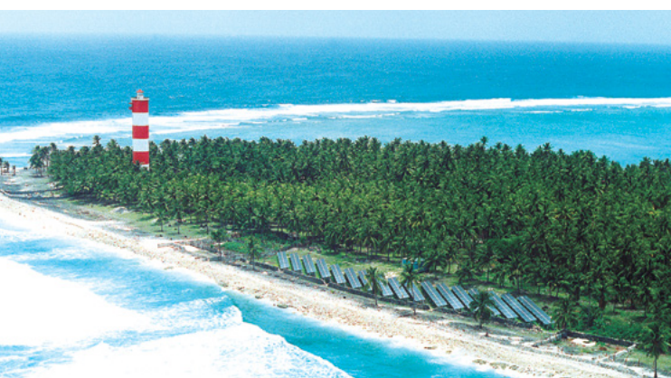
100 kW Grid-interactive Solar PV Plant at Lakshadweep
