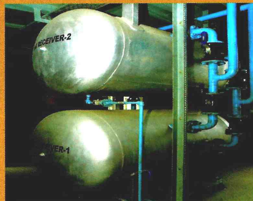
COMPRESSOR UTILITY HOUSE
